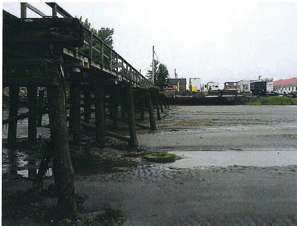
8B: View Looking South of Pile-supported Pier
