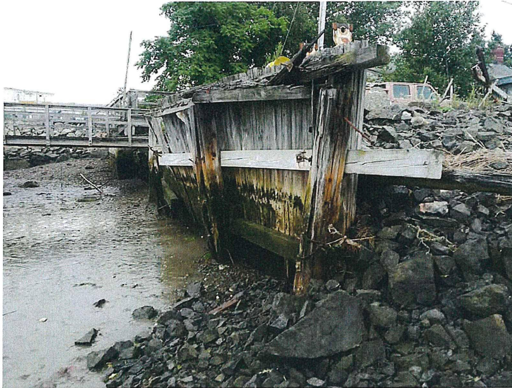
8A: View Looking East near Abutment of Pile-supported Pier
