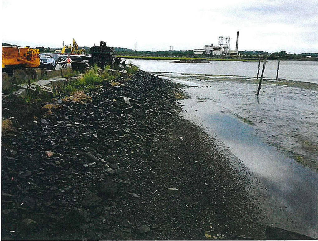
9A: View Looking West along Coastal Bank
